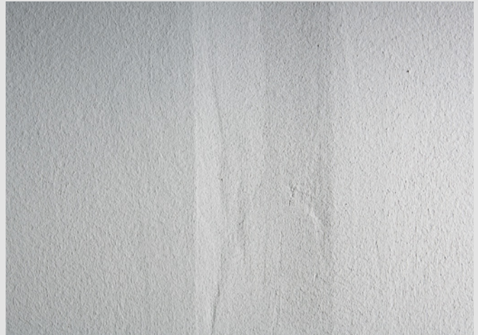
Recessed filled joint with strong side lighting
