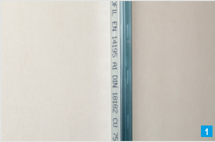
1 Install the profile on the flanking constructional component
