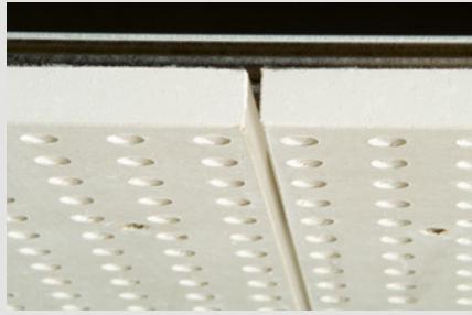
4-side square edge with 3 – 4 mm clearance
