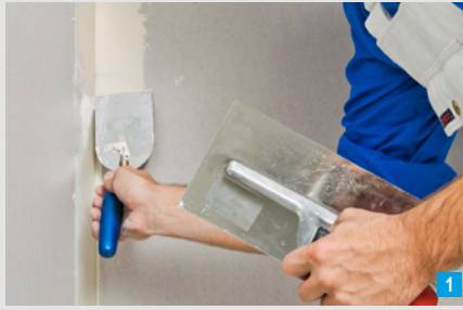
Apply jointing compound
