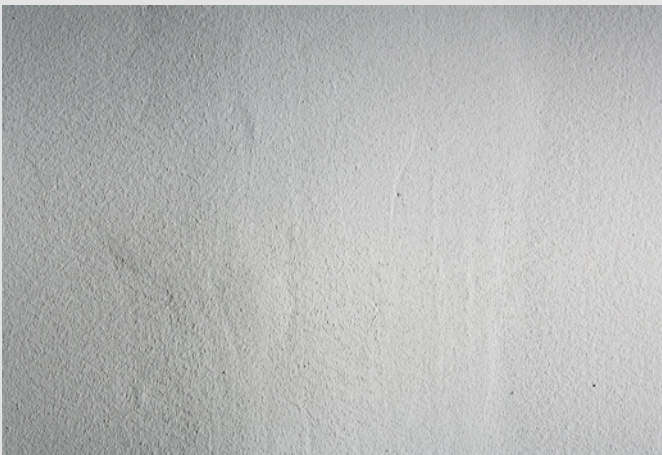
Raised filled joint with slight side lighting
