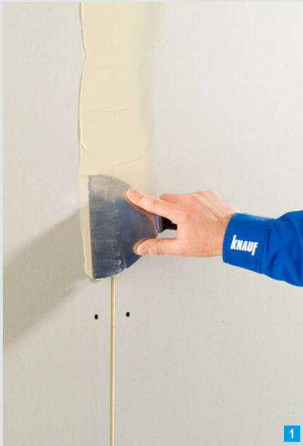
Pressing in of jointing compound
