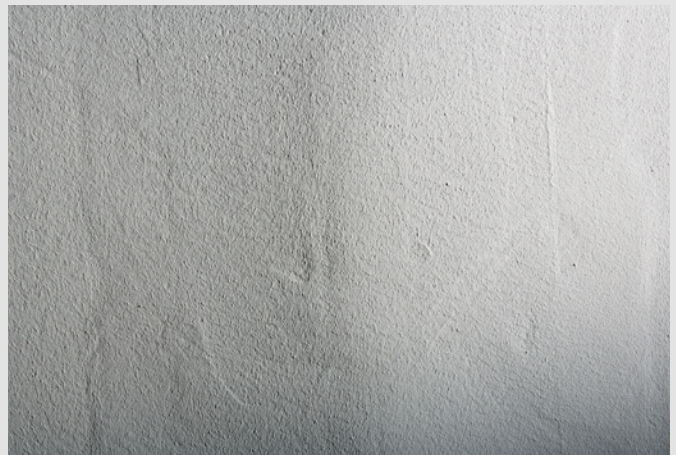
Raised filled joint with intense side lighting
