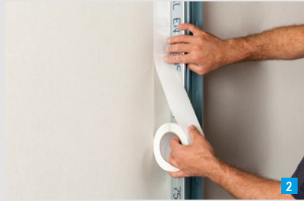
2 Attach Trenn-Fix beside the profile
