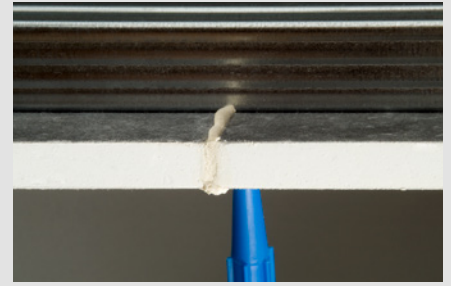
Side view when filling the joint with Knauf Uniflott
