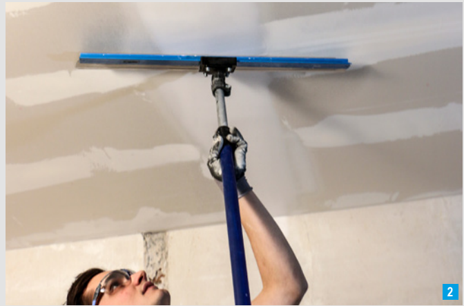
Machine application can achieve up to 5 times greater area coverage.
