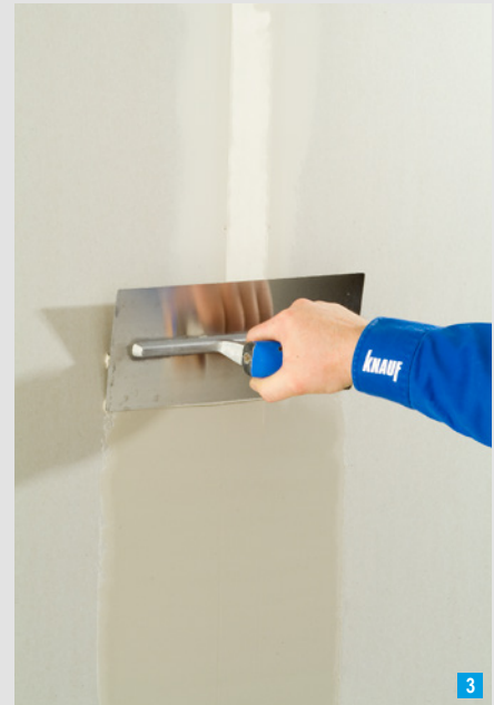
Covering the joint tape with compound using a curved trowel
