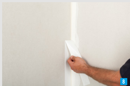
8 Remove the excess strip
