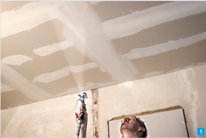
Knauf Fill & Finish can also be applied with airless machines. Simply add one litre of water to a 20 kg bucket.
