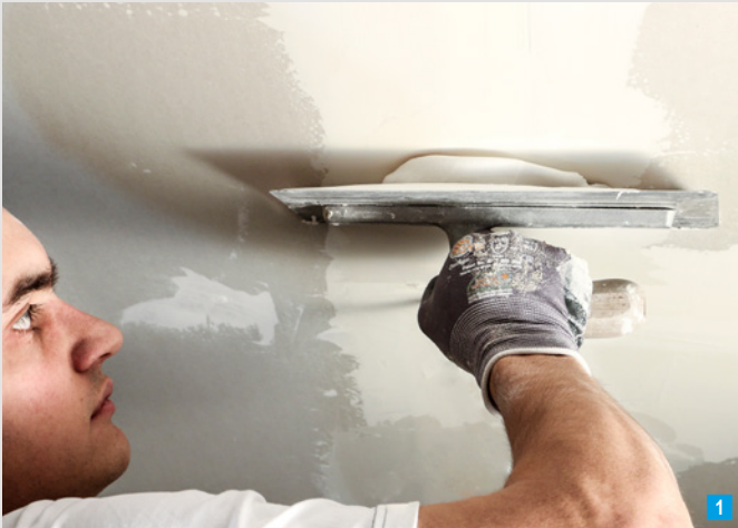
Manual application is possible not just with a finishing trowel, but also using a long pile lambskin roller.
