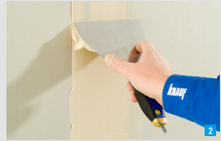
Strike off in longitudinal direction
