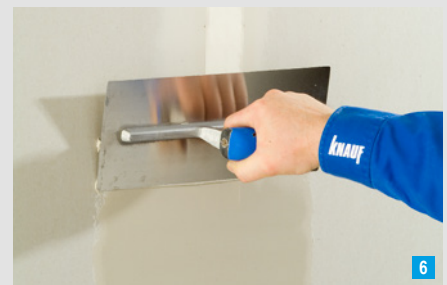
Covering joint tape with compound
