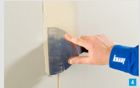
Pressing in of jointing compound
