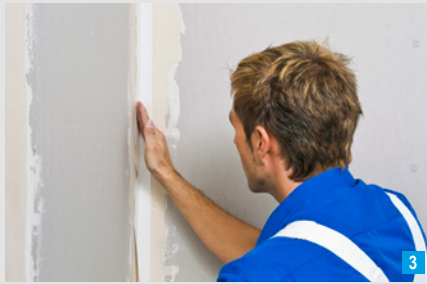
Apply the Knauf Kurt joint tape
