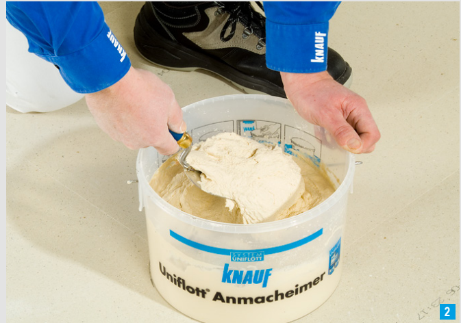
Mixing Knauf Uniflott with a trowel
