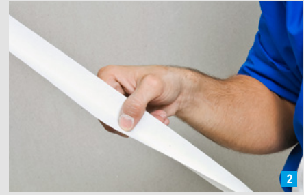
Fold Knauf Kurt joint tape
