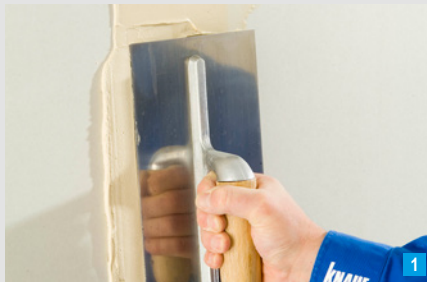
Pressing in of jointing compound perpendicular to joint
