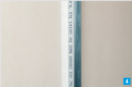
4 Push on the Trenn-Fix and smooth it
