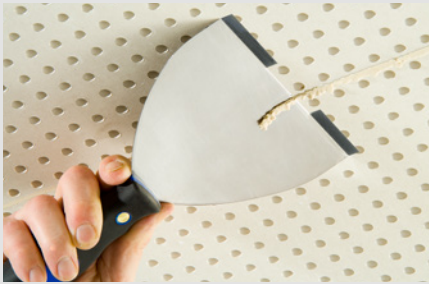
Removal of excessive Knauf Uniflott after drying using the Cleaneo trowel
