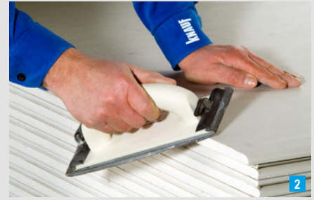
Breaking with the hand sander with Knauf Cleaneo boards
