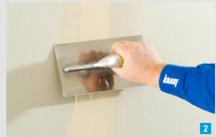
Strike off in longitudinal direction
