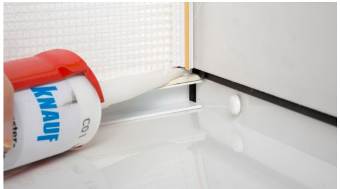
Figure 18: Sealing the interface gap
