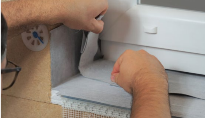
Figure 12: Gluing of the window connection membrane with window sealing membrane
