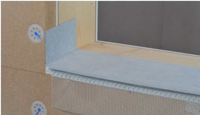
Figure 7: Completed gluing of the window sealing membrane
