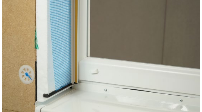
Figure 17: Installation of the window connection profile
