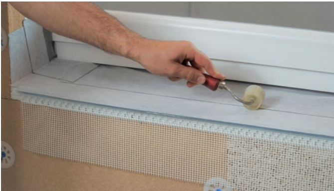
Figure 12: Gluing of the window connection membrane with window sealing membrane
