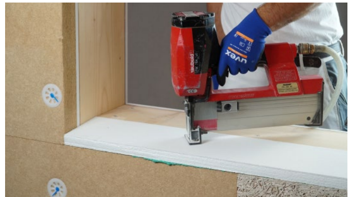
Figure 4: WARM WALL tapered insulation mechanical attachment
