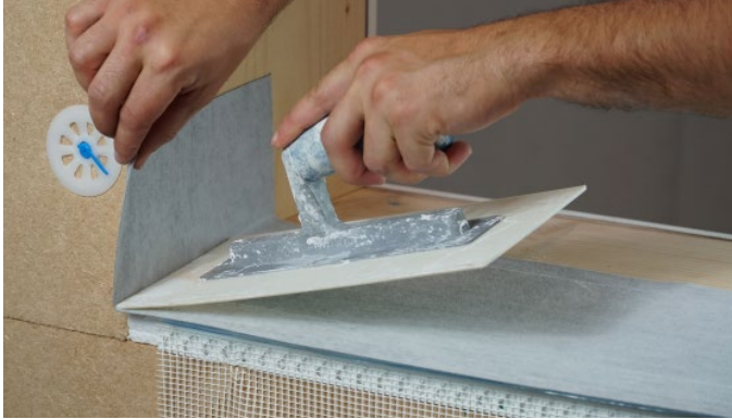
Figure 7: Completed gluing of the window sealing membrane
