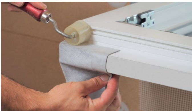
Figure 8: Gluing of the window sealing corner
