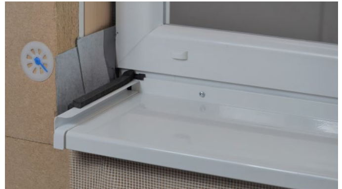
Figure 14: Generous application of adhesive on the window sill
