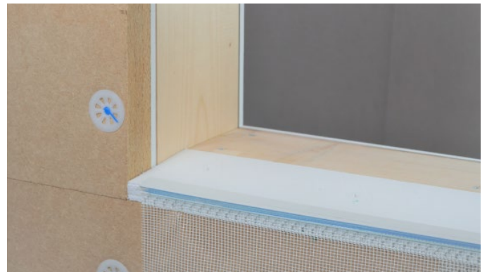
Figure 5: Balustrade profile installation
