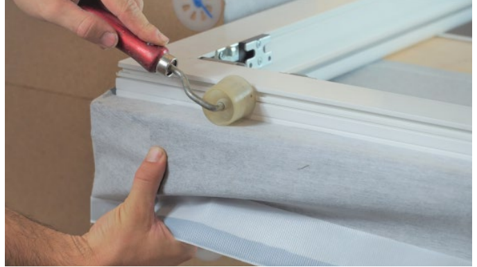
Figure 9: Gluing of the window connection membrane
