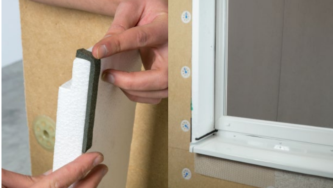
Figure 16: Glued reveal board
