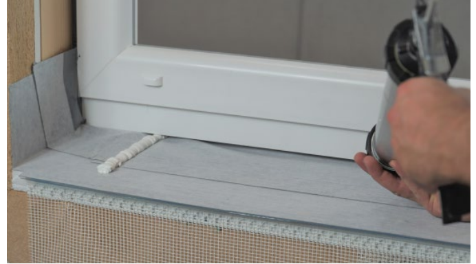
Figure 14: Generous application of adhesive on the window sill
