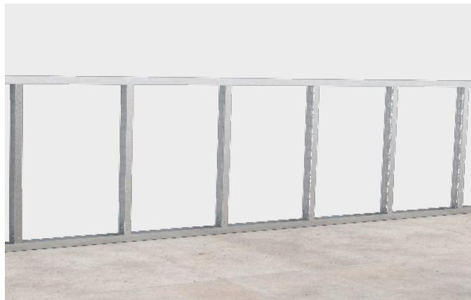
Push on the UW runner and ensure correct alignment.
