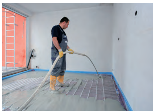
Uponor's Classic system is laid on Knauf's heat insulation and later covered by the self-levelling floor screed FE 50 Largo.
