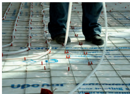
The laying of the sturdy Uponor PE-Xa pipes for radiant temperature control is quick and economical.
