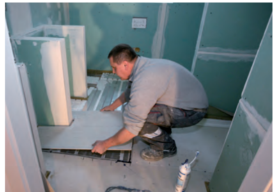
Quick laying of Knauf's Brio Pre-fab Screed on top of Uponor's Siccus panels
